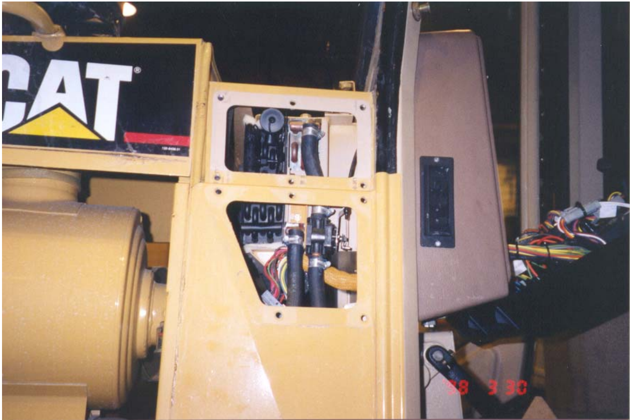
Evaporator in place alongside heater coil.
